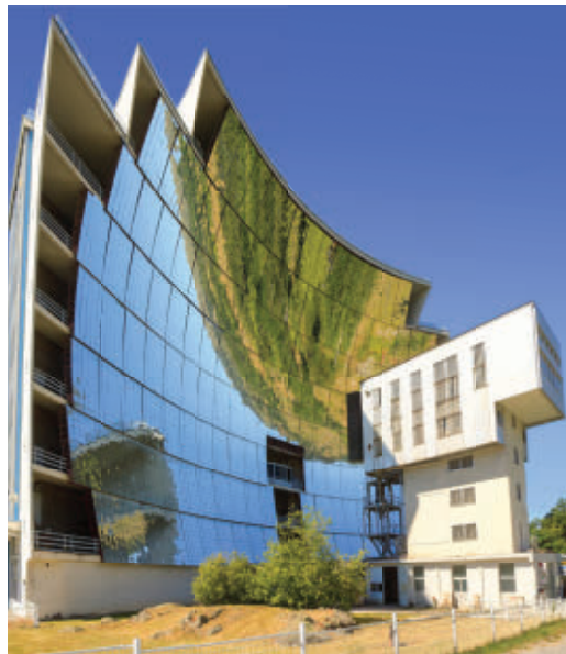
This building-sized curved mirror focuses sunlight into a tight beam and sends it into a vacuum chamber, where the Parker probe’s parts were tested for heat tolerance.
