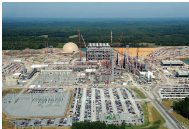
Mississippi's Kemper County CCS facility should open in 2015. The plant will use precombustion capture, turning pulverized lignite into a gaseous mixture, to capture 65 percent of its CO 2 emissions.
