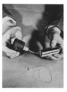
ALTITUDE MEASURED—Carried aloft in balloons, this instrument gives data on altitude by boiling a small quantity of water in the glass vacuum bottle and then measures the water's temperature electrically. The doughnut in the foreground is the heating coil with a tiny battery connected to its wire tail.
